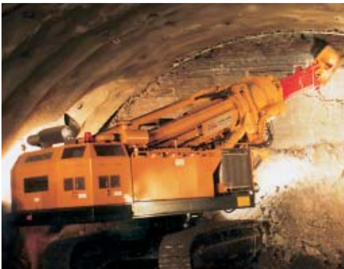
Tunnel profiling with TML Tunneldachs.
