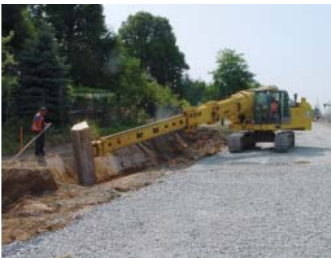
TML boom with extension for extended grading and sloping work.
